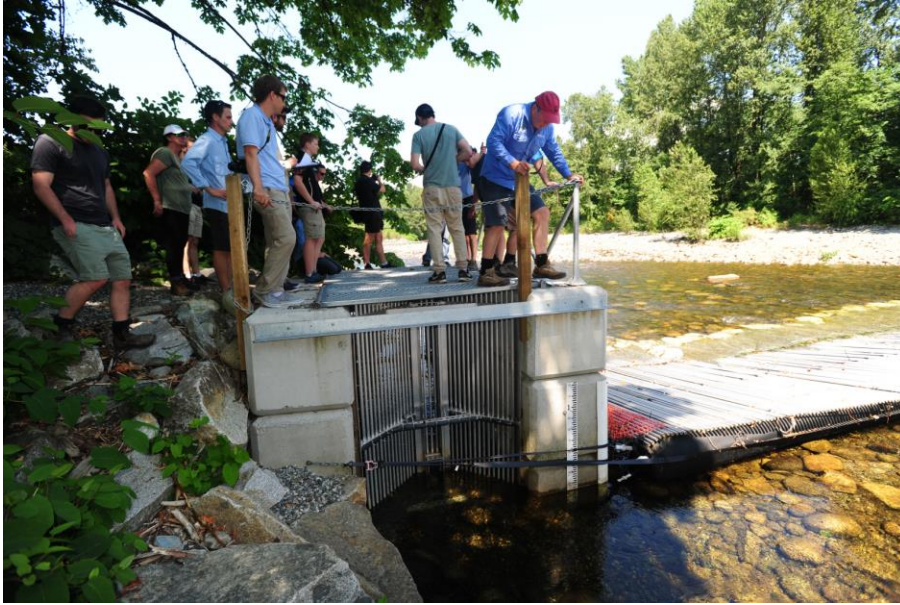
Image 4. Viewing the fish fence and collection gate for capturing returning salmon to be used as brood stock at the Seymour River hatchery.
